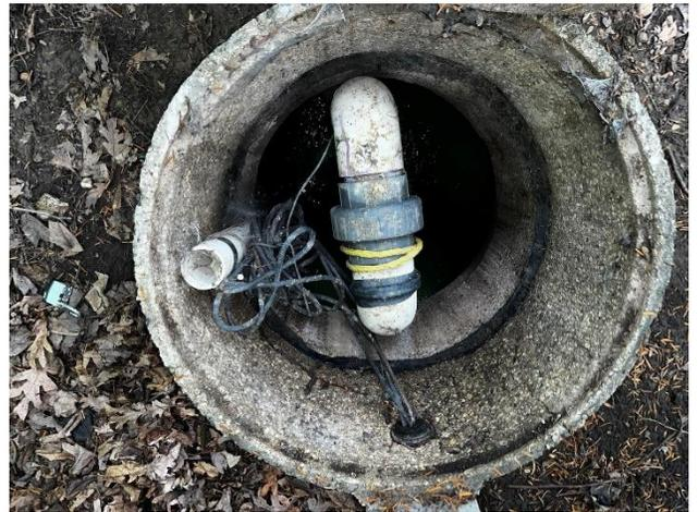
Make sure all manholes are securely replaced and locked for safety. This is so vitally important that I highly recommend either having a line right on your field notes that manhole covers were securely replaced and locked and/or take an 'after' picture of every evaluation you do showing the manhole covers were properly and securely replaced before you left the site.
